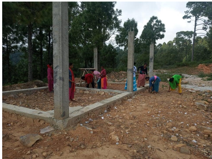
Under constructing CSO's community building - Joroyal 2
